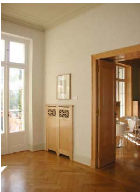
2006, partial views of the restored Living Room showing one original (right) and one reconstructed (left) wooden masks of radi- ators as well as the reconstructed door to the Dining Room.
