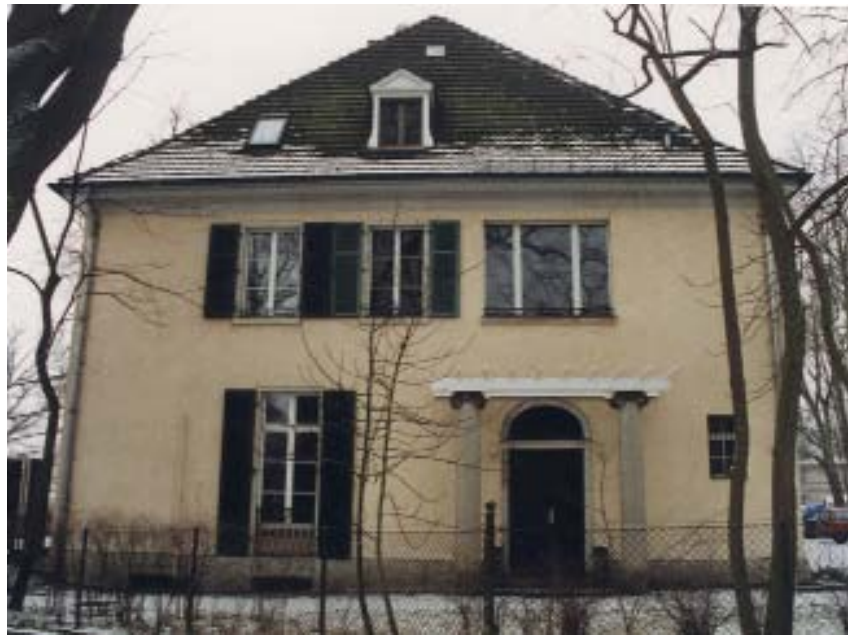
2002, North Façade with coated surfaces
