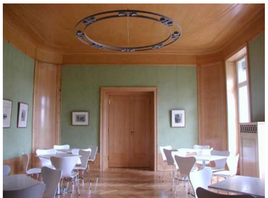
2006, view of the Dining Room's north wall with the restored surfaces and the reconstruction of the double doors.
