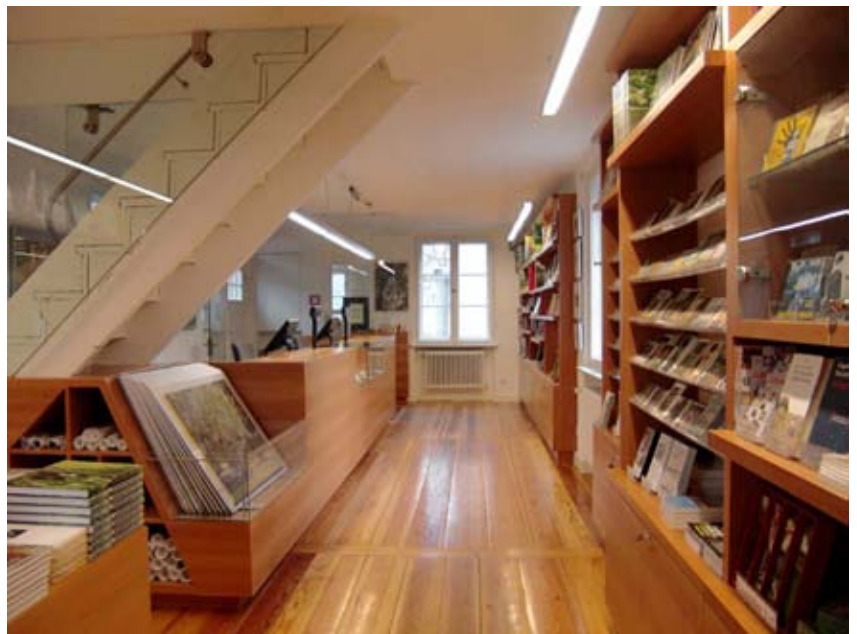
2006, the demolition of the internal walls permitted to create a linear space that serves both as tickets office, information center and Museum Shop.
