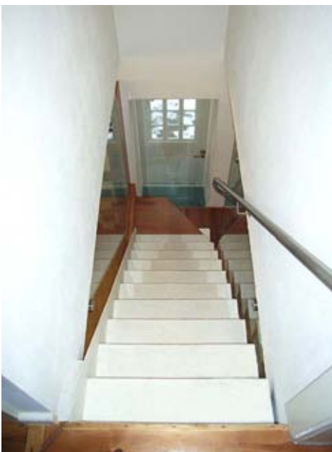
The original wooden stairs remained as a solitary in the middle of the room, the diversion of the lowest steps was accentuated by the use of the same wood as all contemporary shop furniture.
